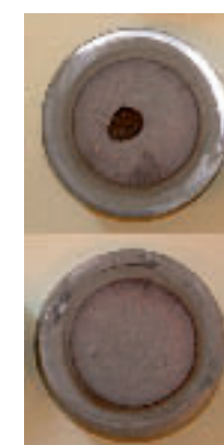
Figure 5 Scabbing of a standard coating with low permeability (top) compared with RHEOTEC XL+ (bottom)
